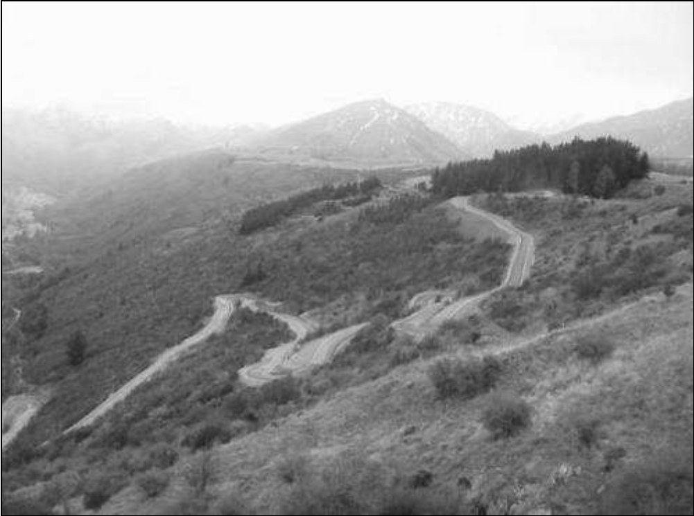
Figure 3 – Looking north at the completed project
