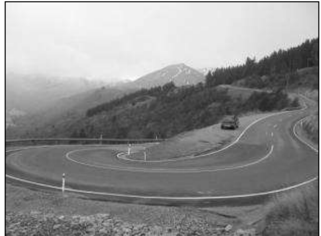
Figure 5 – One of the hairpins after construction
