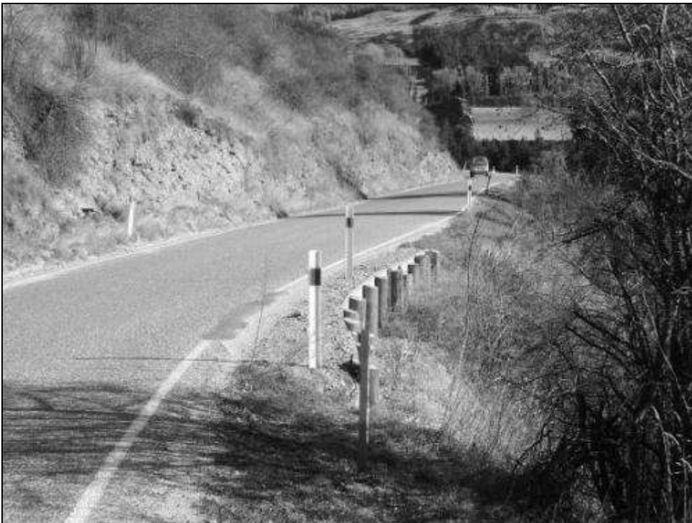
Figure 1 – Looking south along the bottom straight prior to the project commencing
