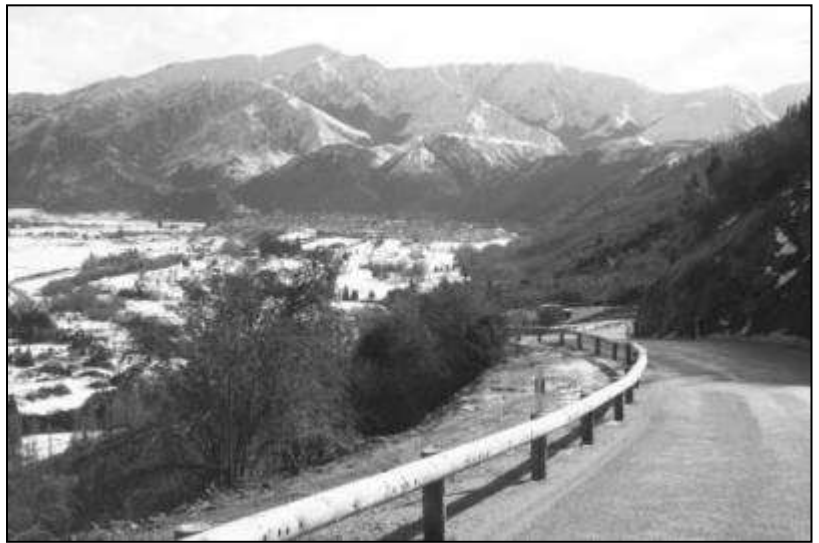
Figure 2 – The completed guardrail
