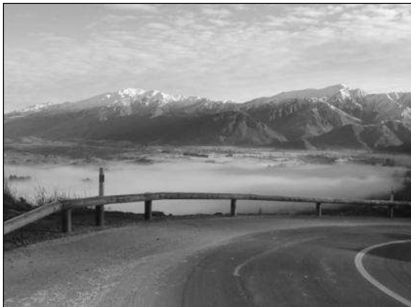
Figure 10 – The timber rail blending into the natural beauty of the area
