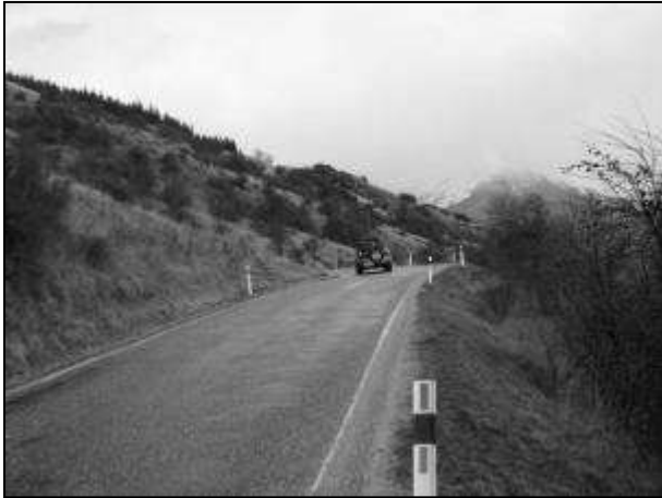
Figure 6 – Prior to construction
