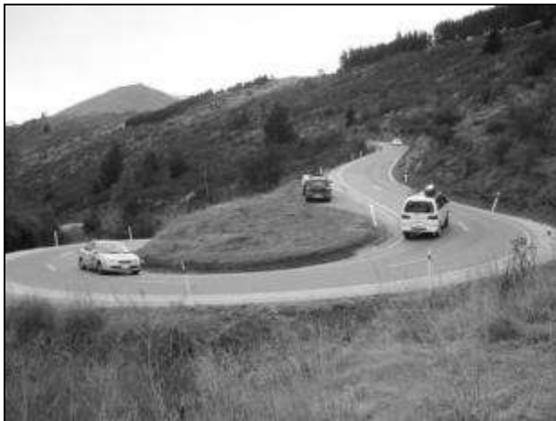
Figure 4 – One of the hairpins before construction
