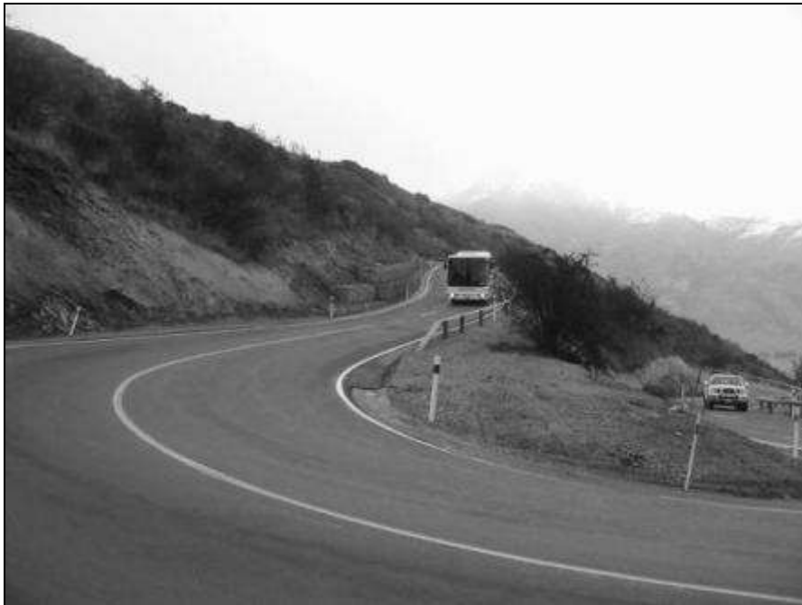
Figure 9 – The road now more safely accommodates large and small vehicles, with room for manoeuvre around the hairpin curves
