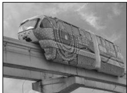
Figure 15: Kuala Lumpur Monorail. Note electrical 'pick up' rail in the foreground on left.
