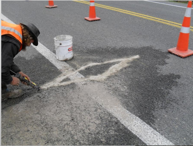
Installation of loops
