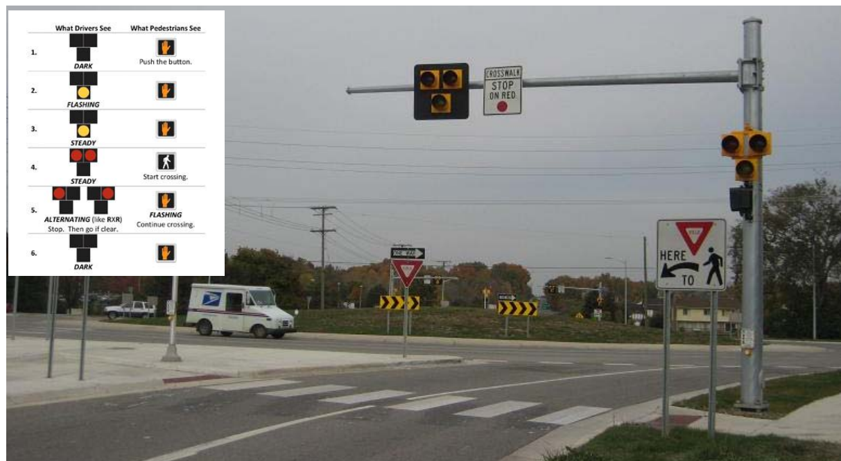
Figure 3: a Hawk signal at a two-lane entry to a roundabout in Michigan, the United States. The HAWK can optionally be set up so pedestrians have the discretion of either crossing the road as at a regular zebra crossing or push the button to call up the signal phase.
