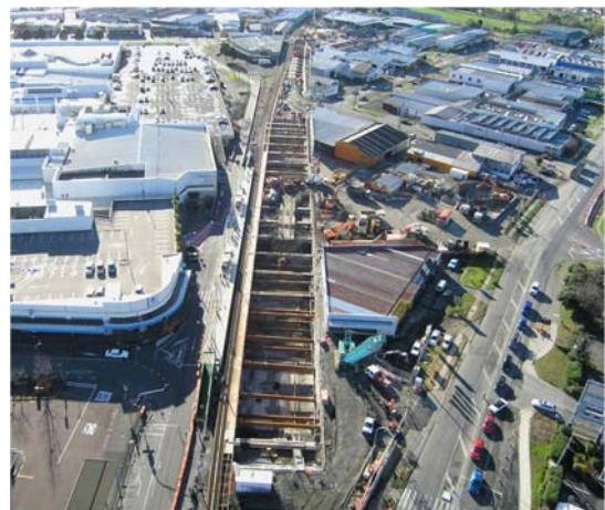
Figure 1: New Lynn Rail Trench under construction
