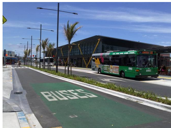
Figure 3: Constructed "Enhanced Station" with wrap around bus facilities
