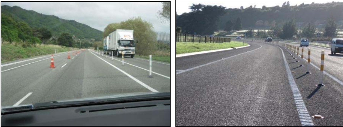
Figure 1. Peka Peka passing lane southbound (left) and northbound (right) with safe-hit post median treatment.
