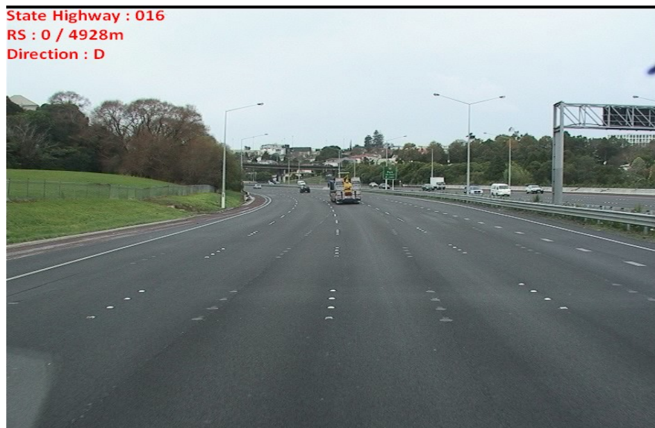
Photo 2: Example from Auckland Motorway
