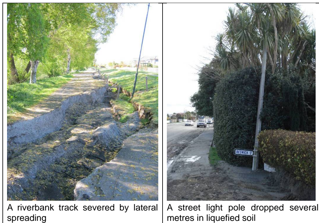
Figure 1: Photographs of earthquake damage in Kaiapoi
