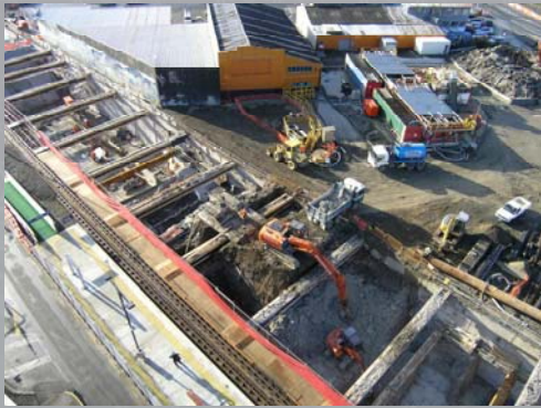
Stage 3 – Prop and dig
