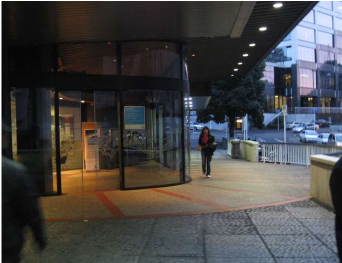
Network cameras installed inside the central library
