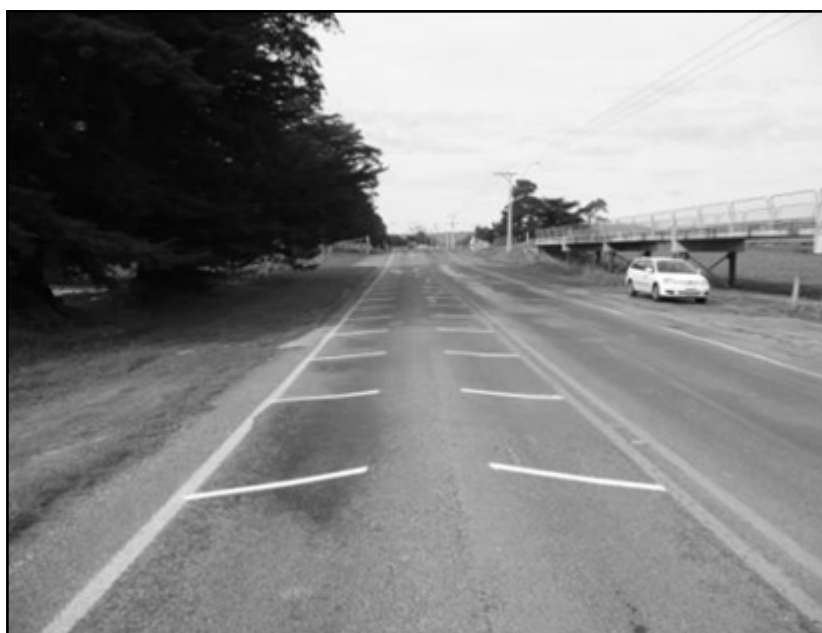
Figure 7: Established SH53 trial site (410m from the bridge hazard)
