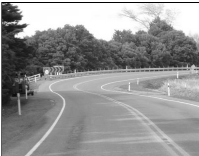
Figure 6: Eastbound approach to the SH53 trial site (50m from the bridge)
