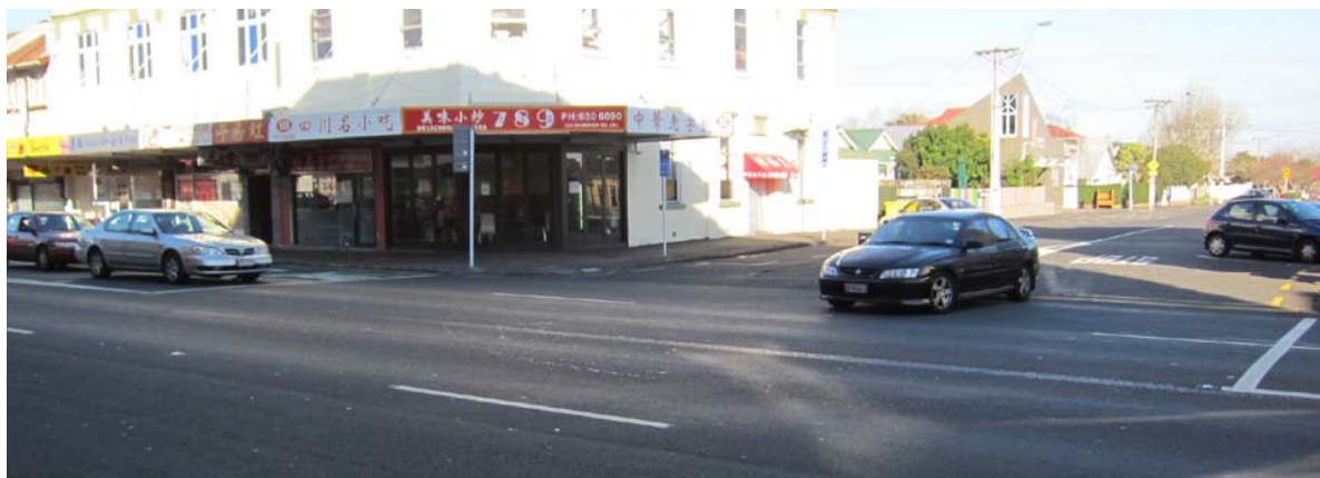
Figure 7 – Wiremu St/Dominion Rd intersection, showing holding lines to encourage better queuing behaviour
