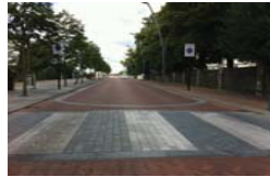
Use of double "kerb" to visually narrow the carrieway in Ashford, Kent
