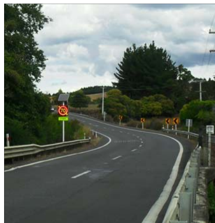
SH27 Southbound April 2013
