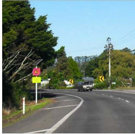
SH25 Southbound April 2013
