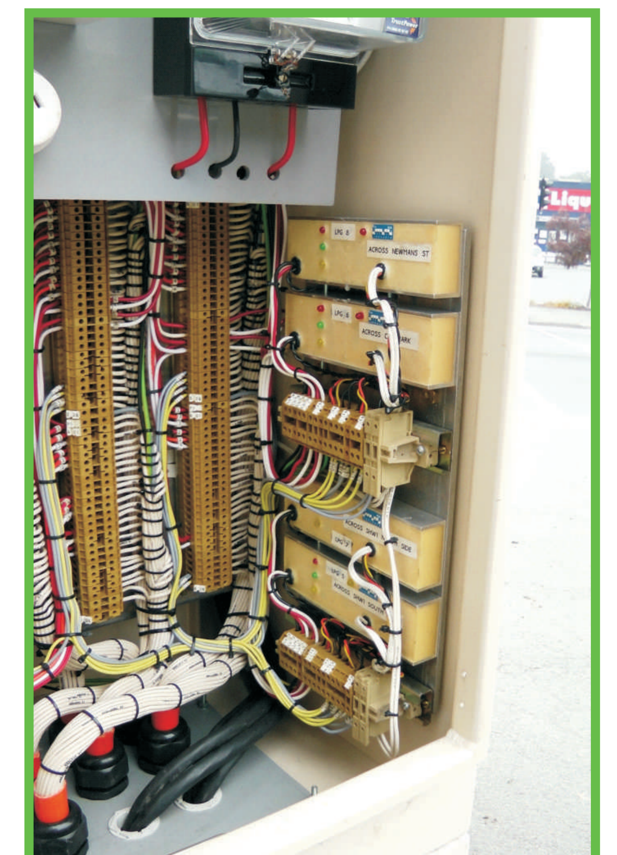
Figure 3: Photo showing four beige DPCS driver units in a controller unit.
