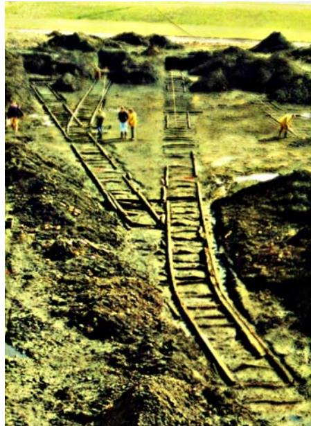
Lambton tramway being excavated and recorded, 1997.
