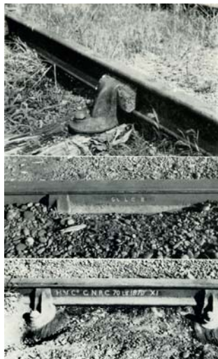
Inappropriate standards for New Zealand, 1860s. Still in use, 1963.
