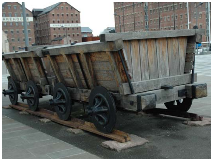
Wagons for the 3'-6" gauge Gloucester & Cheltenham tramway of 1805. Plain wheels running on flanged cast iron rails.
