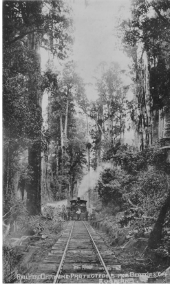
Developing the central North Island - Ohakune railhead, 1908.
