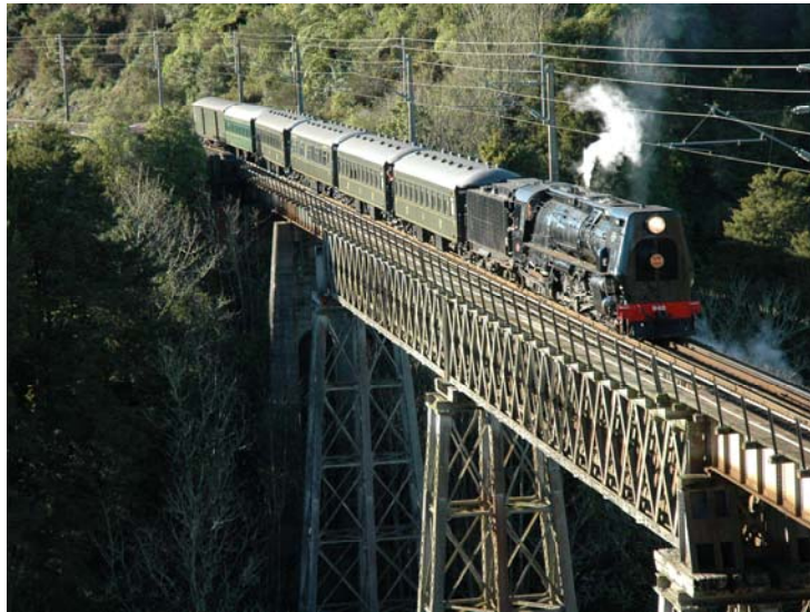
Waiteti viaduct, North Island Main Trunk Line, built by Andersons Ltd 1887-8.
