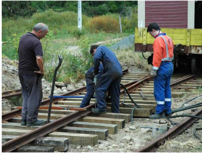
A heritage railway track gang building a turnout.
