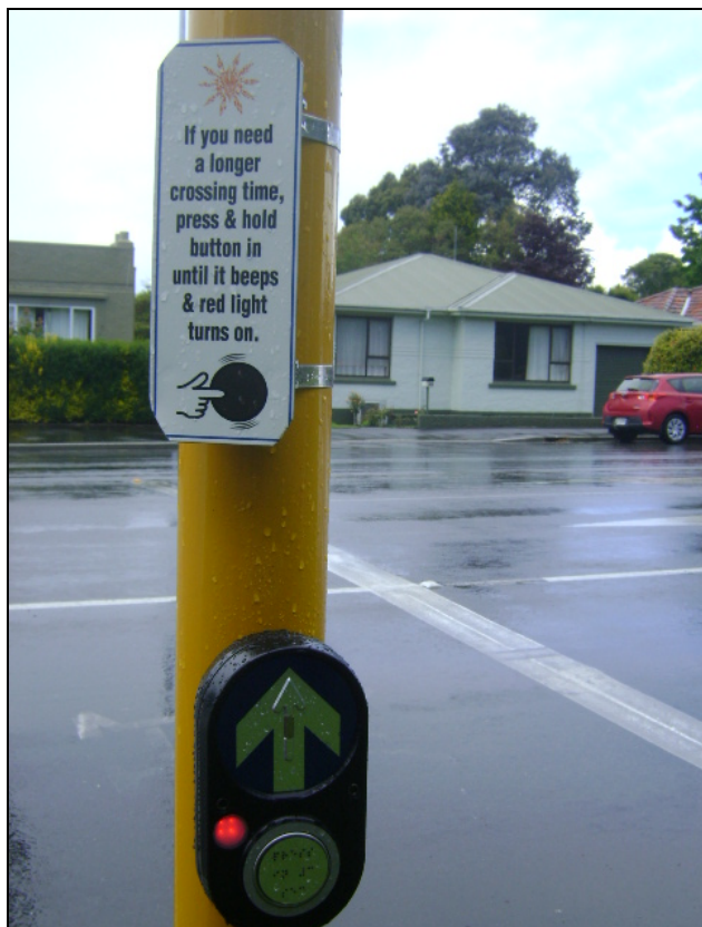
Figure 5 - DPCS Signage and call unit with red LED activated, advising pedestrians that longer crossing time has been chosen
