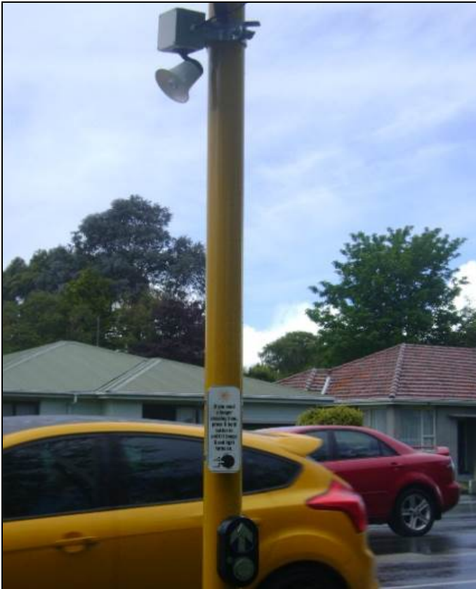
Figure 1 - Integrated DPCS Trial Hardware showing audible voice message unit, signage and new pedestrian call unit with red LED and braille label
