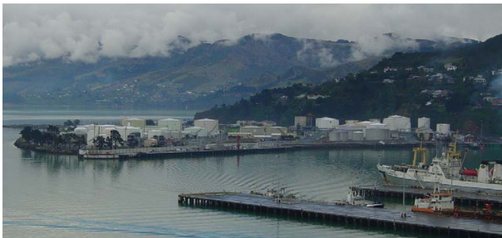
Figure 3 Petroleum Bulk Storage Facility at the Port of Lyttelton
