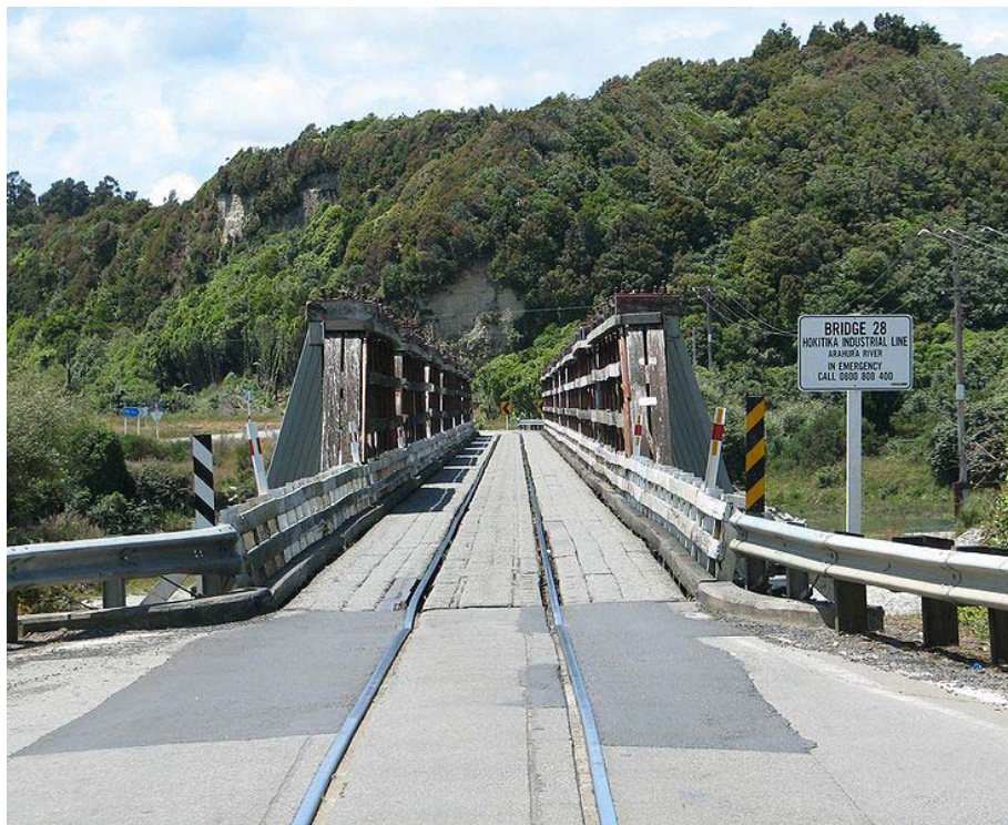
Figure 3 SH6 Arahura Bridge – multifunctional structure
