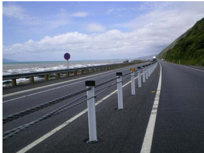
Figure 5 SH1 Centennial Highway, Wellington narrow median barrier
