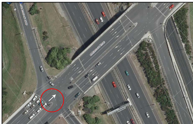
Figure 20: A supplementary straight ahead arrow located immediately in line of sight of a driver stopped at the limit lines.
