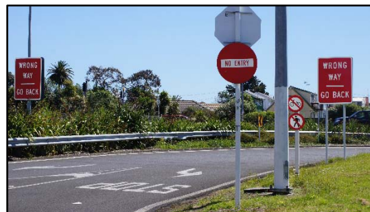
Figure 15: Creating a band of signs, a ‘Sea of Red’ as viewed from the limit line for turning traffic into the off ramp
