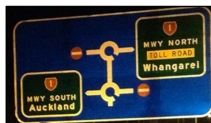
Figure 11: Diagrammatic sign clearly indicating the relative position of the on and off ramp locations
