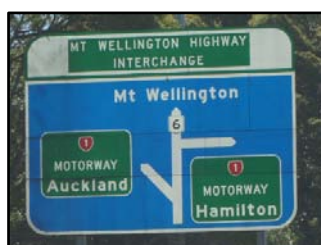
Figure 10: While this sign is uncluttered and hence quick to interpret, it excludes the relative location of the off ramps. This may lead to a motorist entering the wrong ramp.
