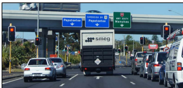
Figure 18: Overhead Lane Assignment Sign giving clear guidance as to which lane to be in. Compared to Figure 16
