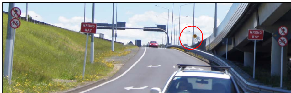
Figure 12: Permanent warning sign for busway visible from off ramp
