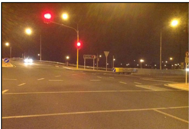
Figure 22: Median barrier hindering conspicuity of the on ramp
