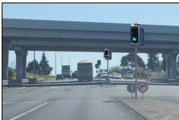
Figure 13: Typical Signals at a diamond interchange
