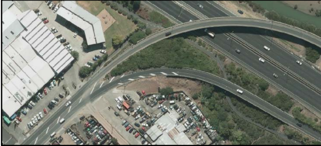
Figure 1: Local road leading to on and off ramps
