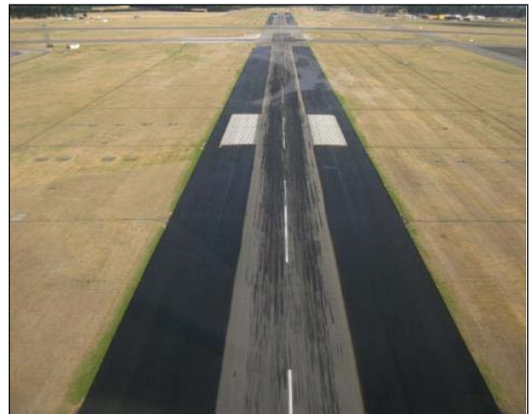
Figure 7: Birds Eye View of Broken GSB-88
