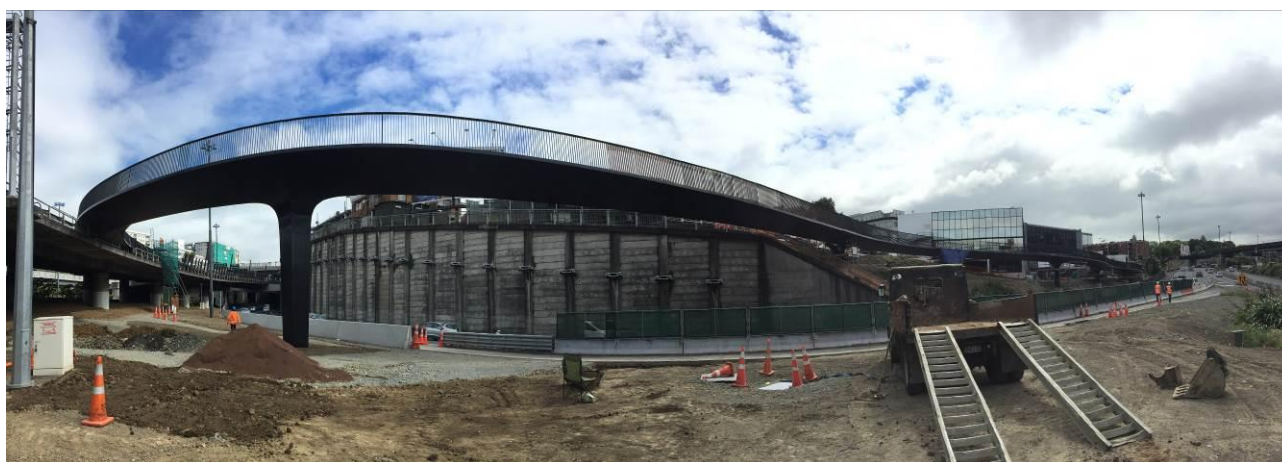
Figure 4 – Bridge Panorama showing bridge continue along embankment (view from SH1 median)
