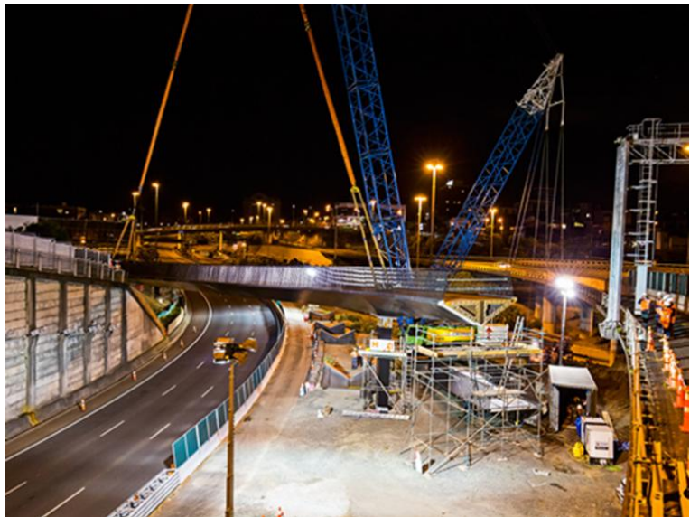
Figure 5 – Beam 2 lift (52m and 95tons)
