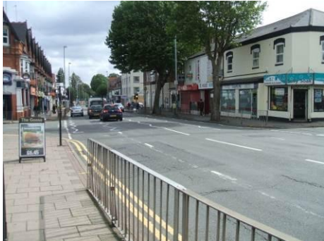
LOCATION 1. Highway dominated environment, wide carriageway with four traffic lanes. Barriers to pedestrian movement.
