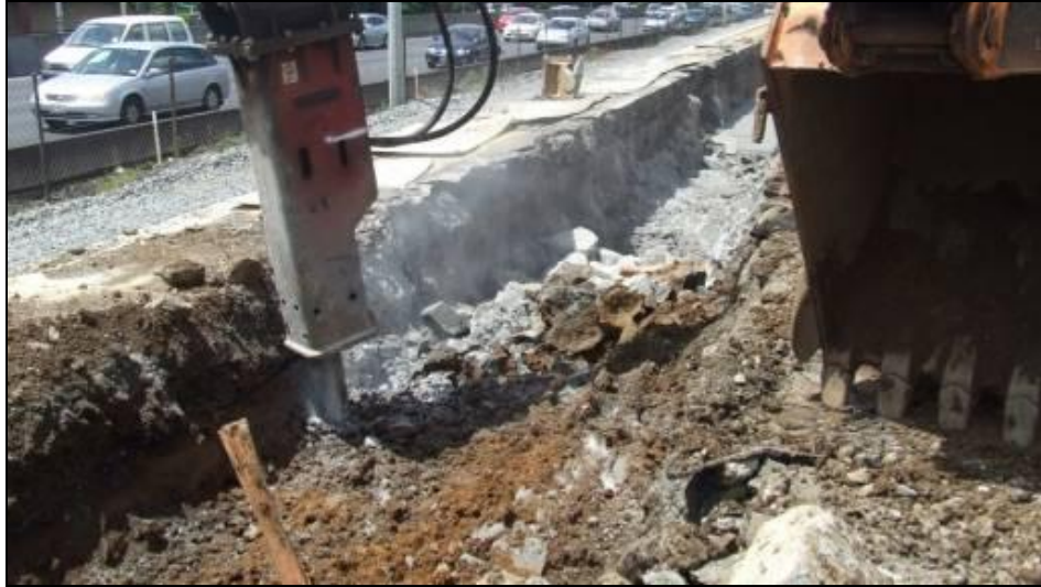
Figure 5: Different ground condition
