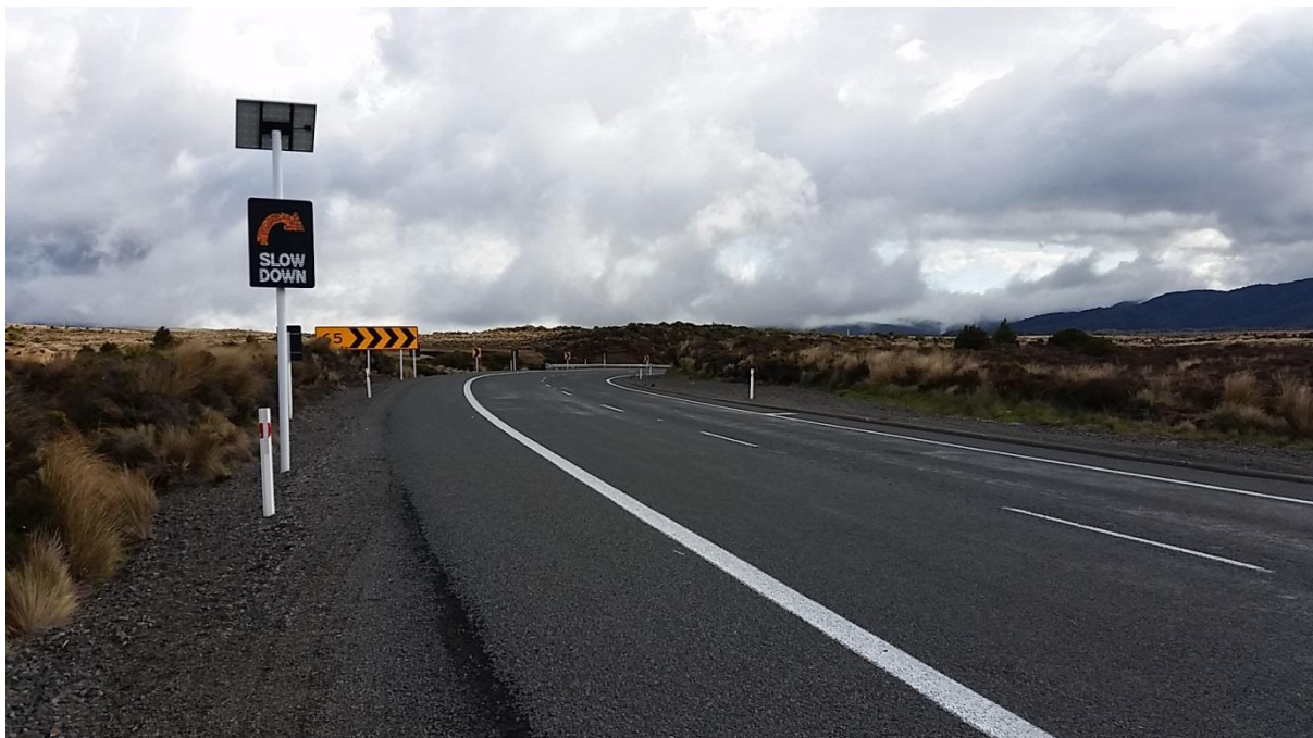
Figure 1: Example of electronic curve warning sign in action (on SH1 Desert Road)
