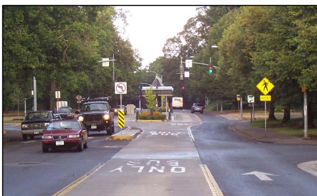
Figure 13: Two-way central bus lane splits at a bus stop, Eugene OR, US
