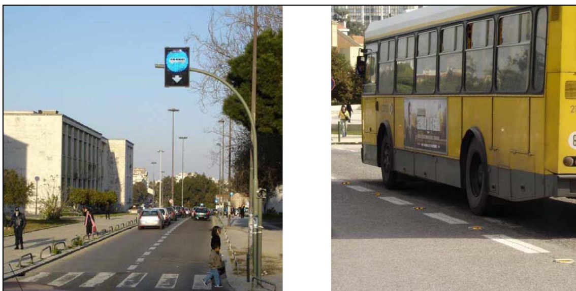
Figure 17: Dynamic signage and in-pavement lights used to indicate intermittent bus lane on Alameda da Universidade, Lisbon, Portugal (Viegas et al 2007)
