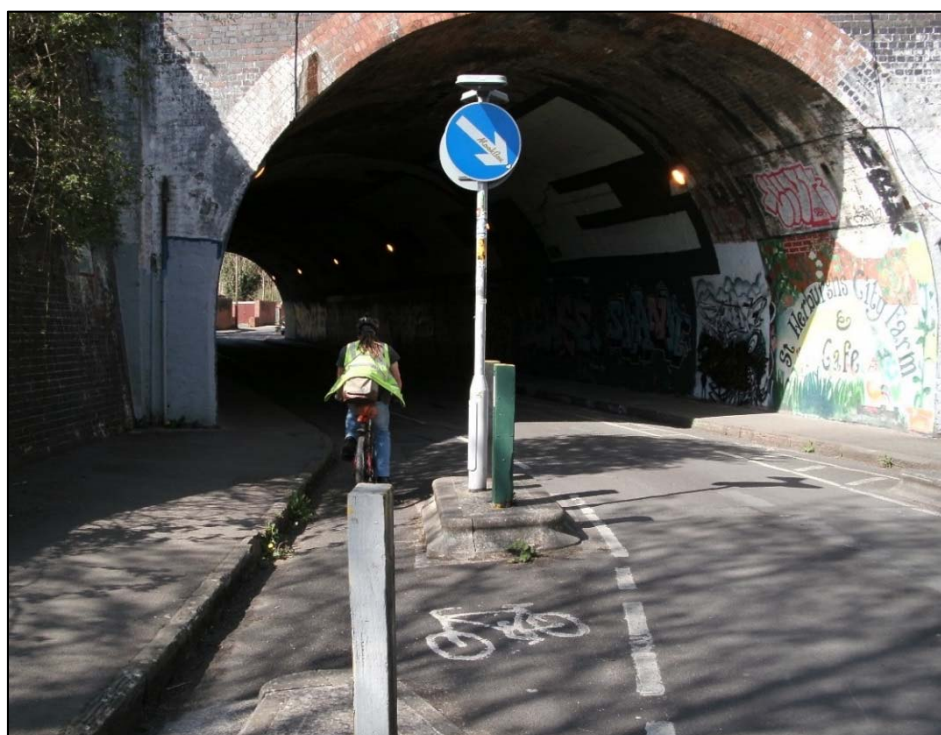
Figure 20: Cycle lanes either side of a single traffic lane, Mina Rd tunnel, Bristol UK
