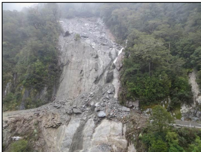
Figure 2: Landslide after the initial event on 10 September 2013
