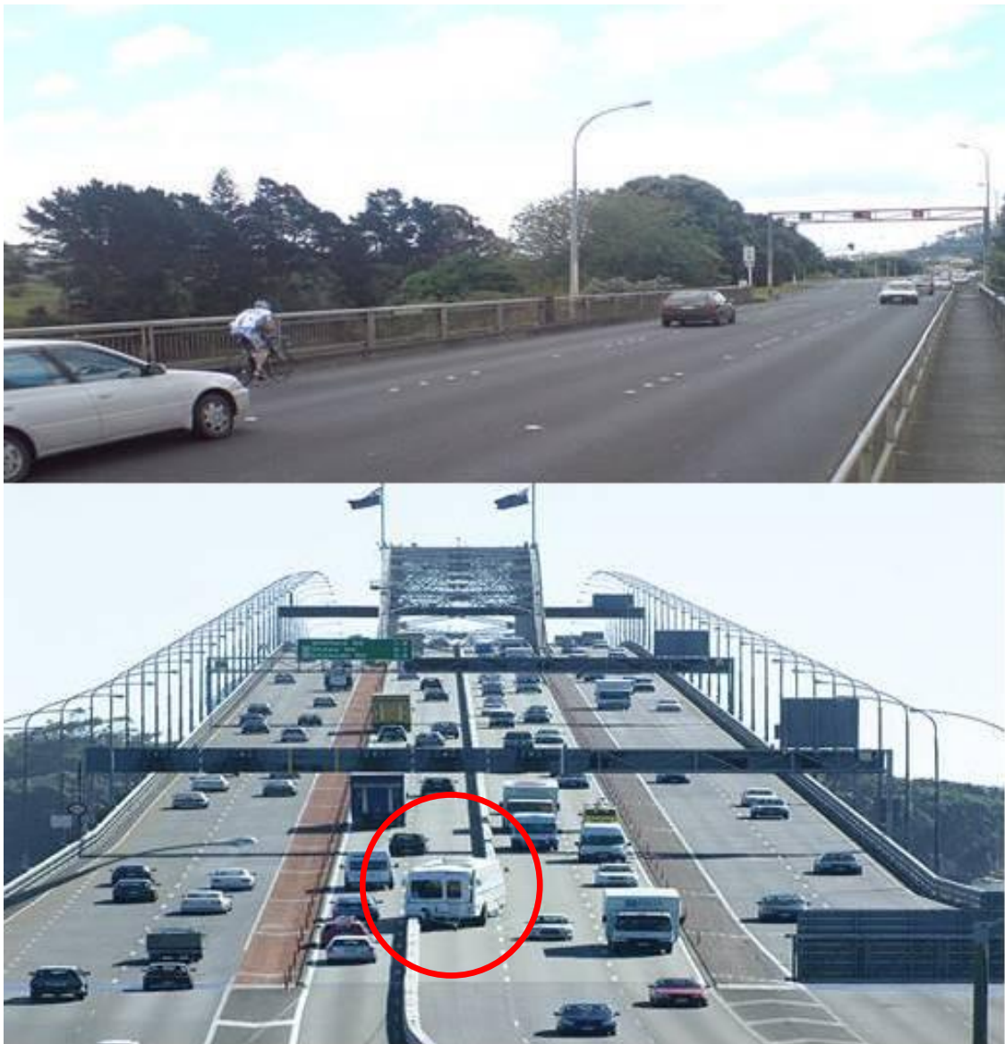
Figure 1: (Top) Panmure Bridge, (Bottom) Auckland Harbour Bridge.
