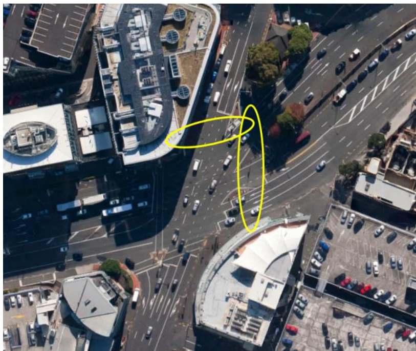
Figure 5: Missing pedestrian crossings at the Sturdee Street / Fanshawe Street / Nelson Street / Market Place intersection
