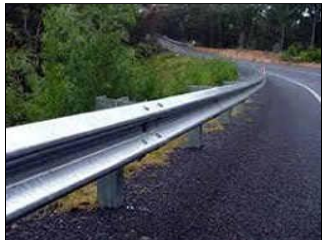
Figure 2 Example of a W-beam barrier
