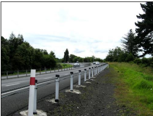
Figure 1 Example of a wire rope barrier
