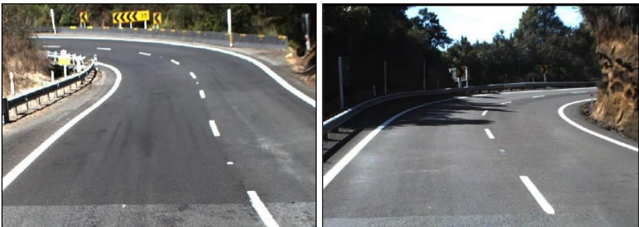
Figure 5 W-beam high incident site #2 SH01N RS 777 RP5900–5910
