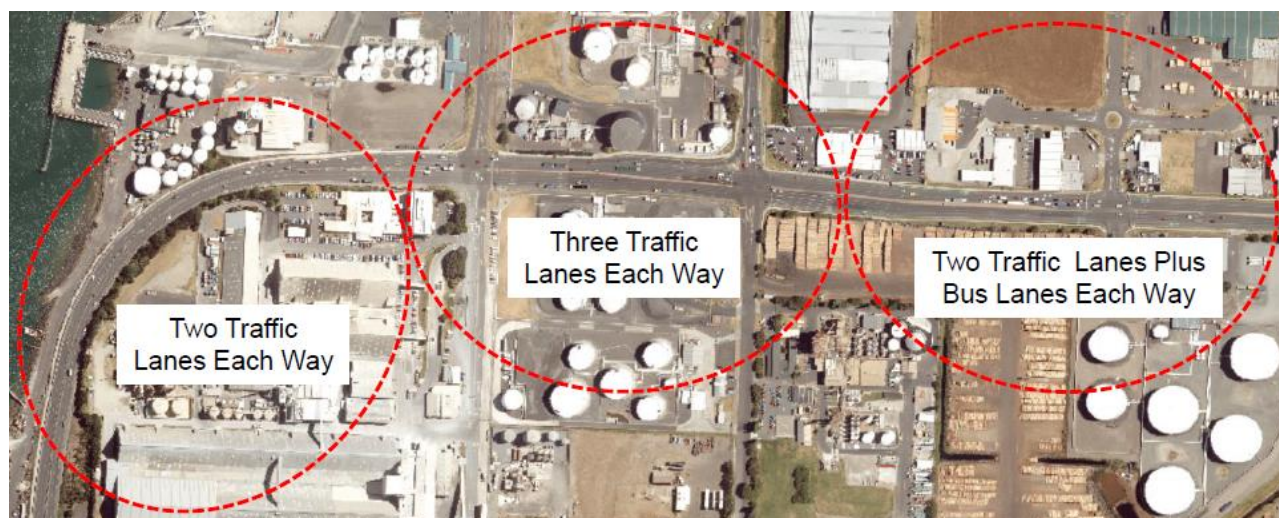
Figure 5: Existing Lane Configuration
