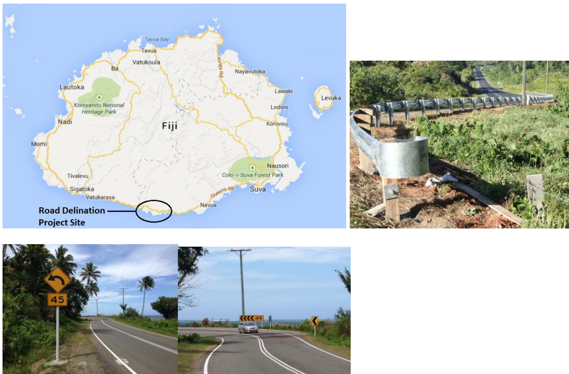
Figure 6: Mass action delineation trial (15km) and safety barrier upgrades
