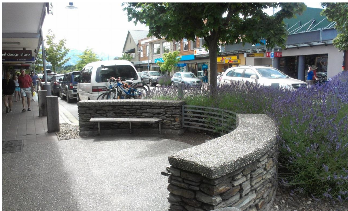
Figure 4: Example of Kerb Build Out between Parking Bays (Wanaka)
