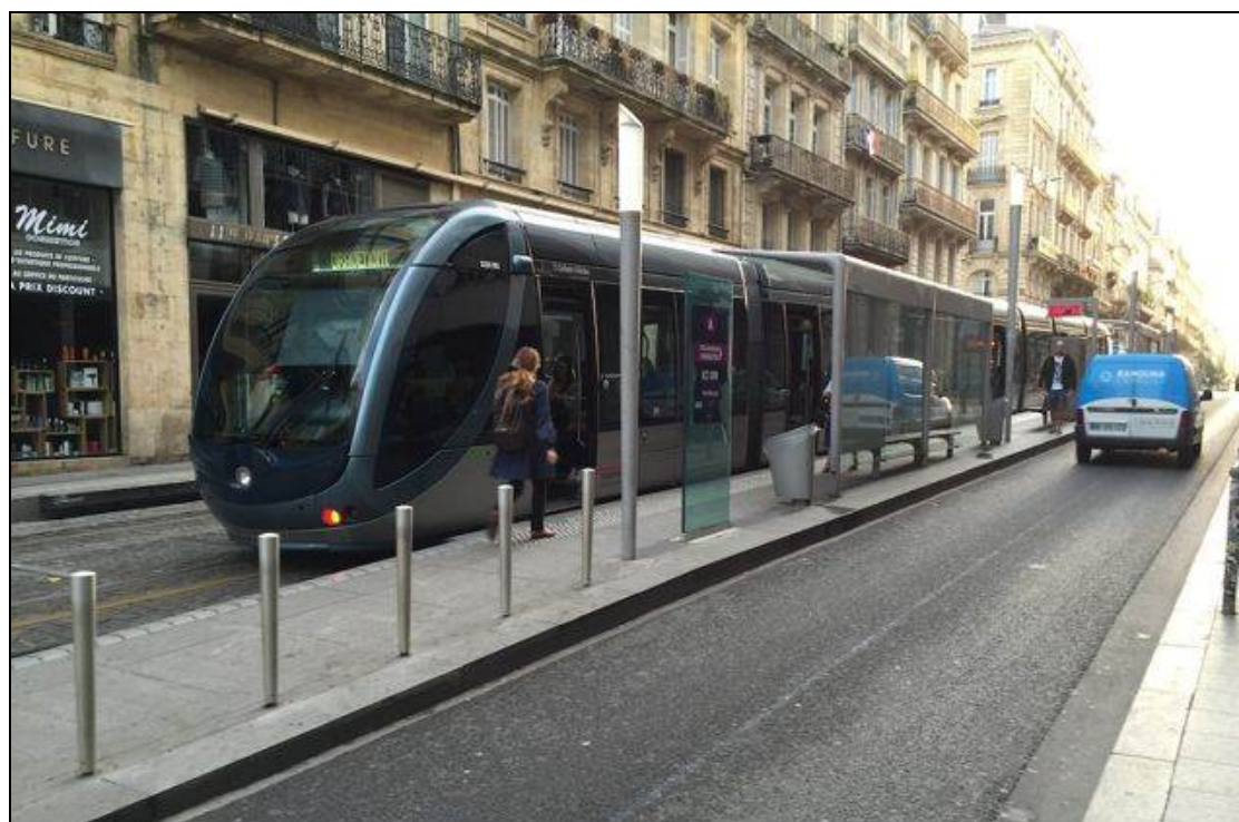
Figure 5 Bordeaux LRT in a narrow street (15m) with a single traffic lane
