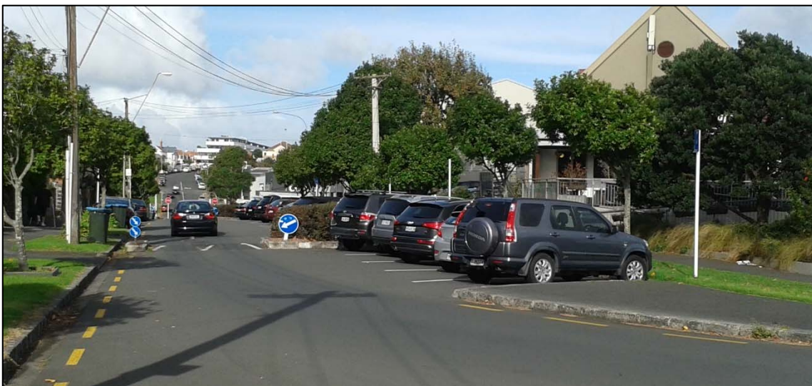
Figure 5: View of Selbourne St looking south (one-way direction)
