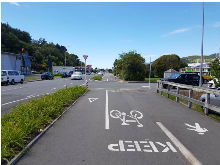
Photograph 4 SCL approach to Parere Street, showing giveaway control
