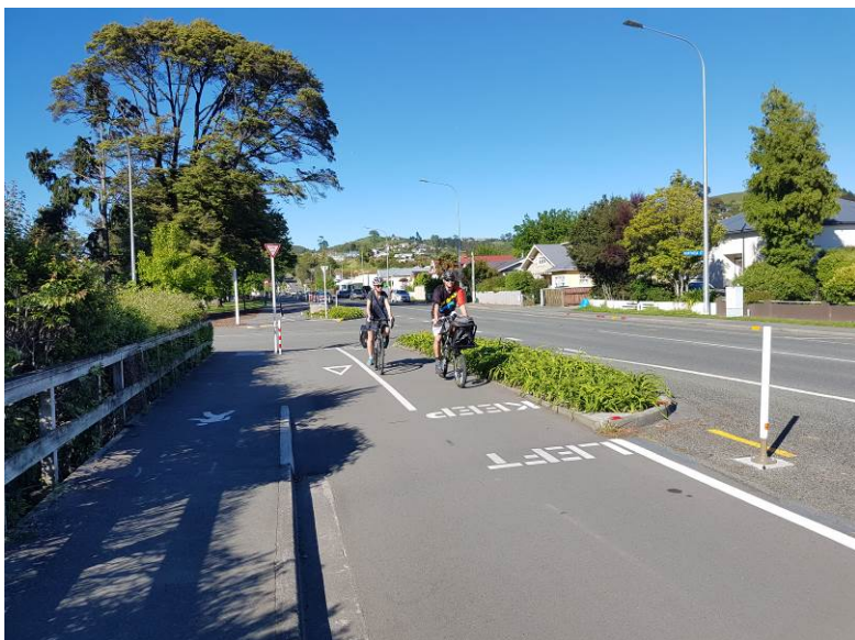
Photograph 1: St Vincent Street SCL Facility near North Esk Street Intersection looking south.
