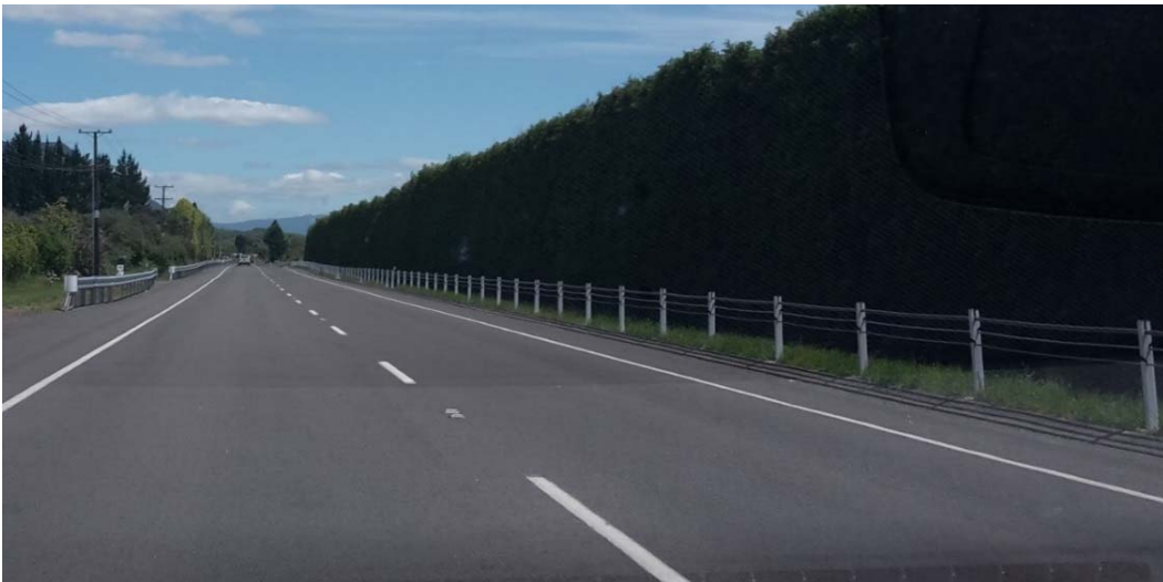
Figure 4 – Photo of side barrier installed on SH30 Te Teko to Awakeri
