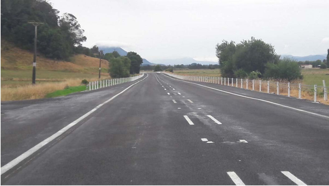
Figure 3 – Photo of side barrier and wide centreline installed on SH30
