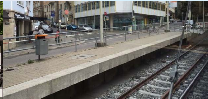
High floor LRT (Stuttgart)
