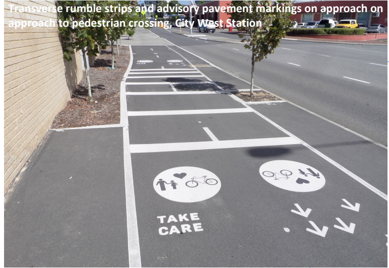
Path deflection treatment on approach to pedestrian crossing, City West Station
