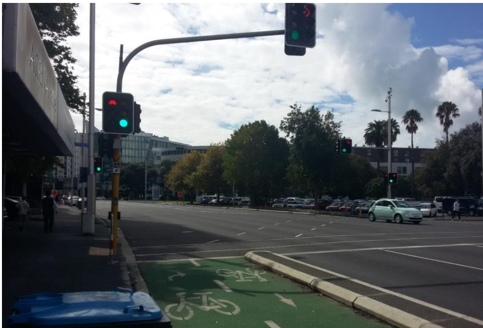
Figure 1: Beach Road diagonal crossing with original signals
