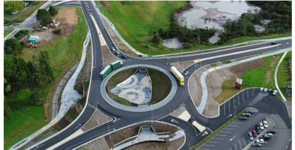
One-off Solutions Hemo Road Roundabout, Rotorua
