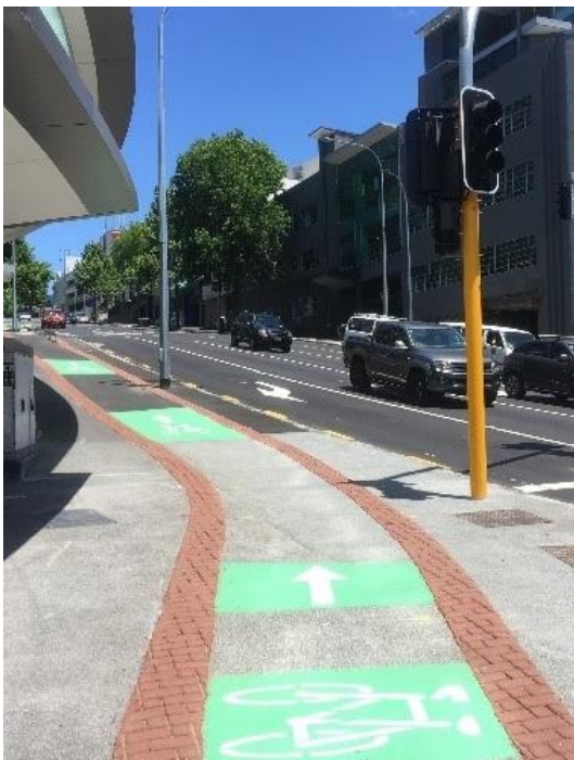
Nelson Street - red thermoplastic 'brick' inprint - 300mm wide, 10-12mm high
