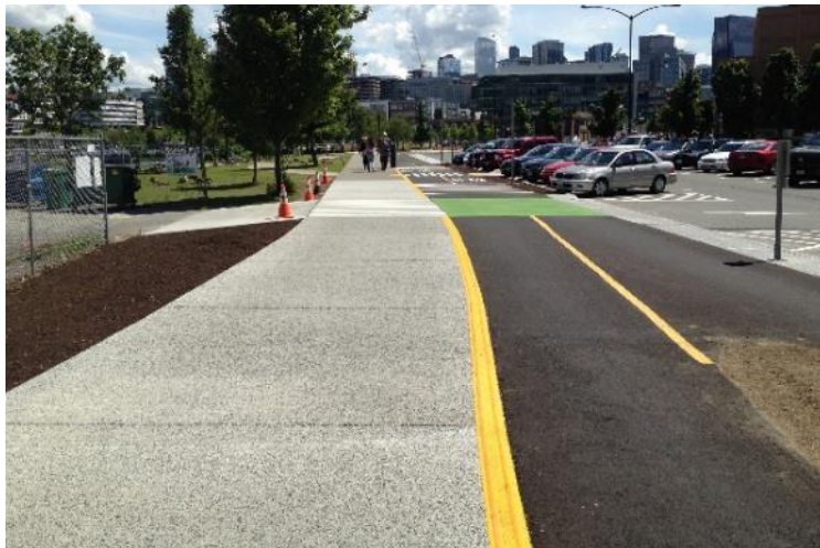
Seattle - 150mm wide, double ridge of 6mm high thermoplastic strips
