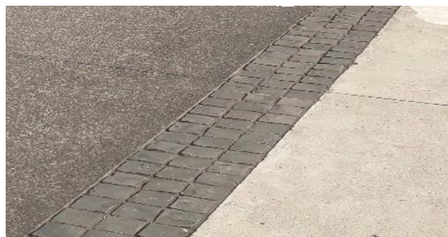
Upper Queen Street - 300mm wide basalt set strip
