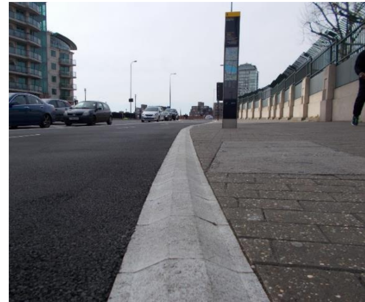
London – 150mm wide – 20mm high concrete
