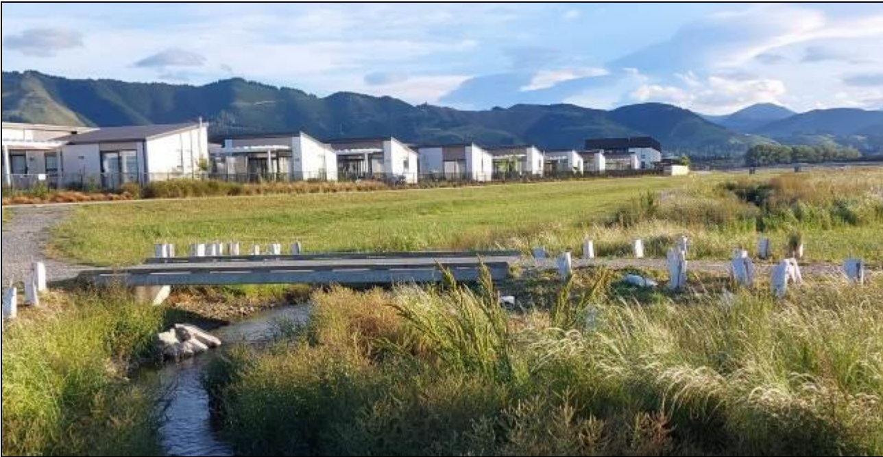
Figure 8: One of the low flow crossings
