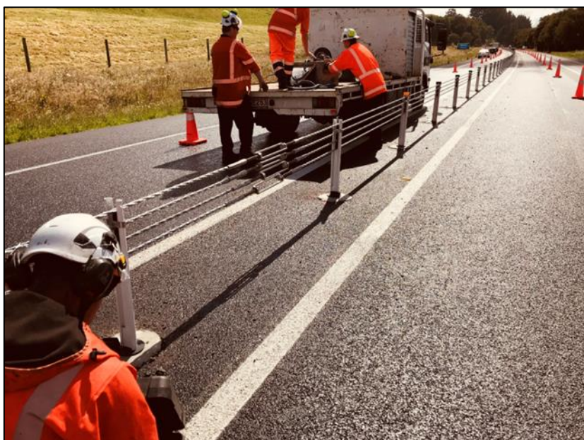
Figure 9 Median Barrier Installation – SH1 Cambridge to Piarere
