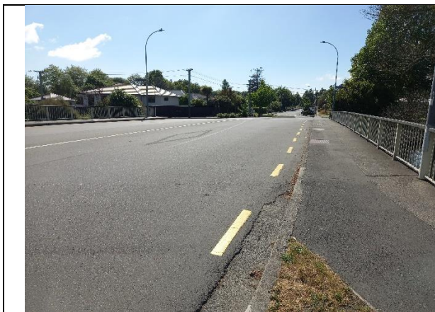
View from the south side looking east (57m)
