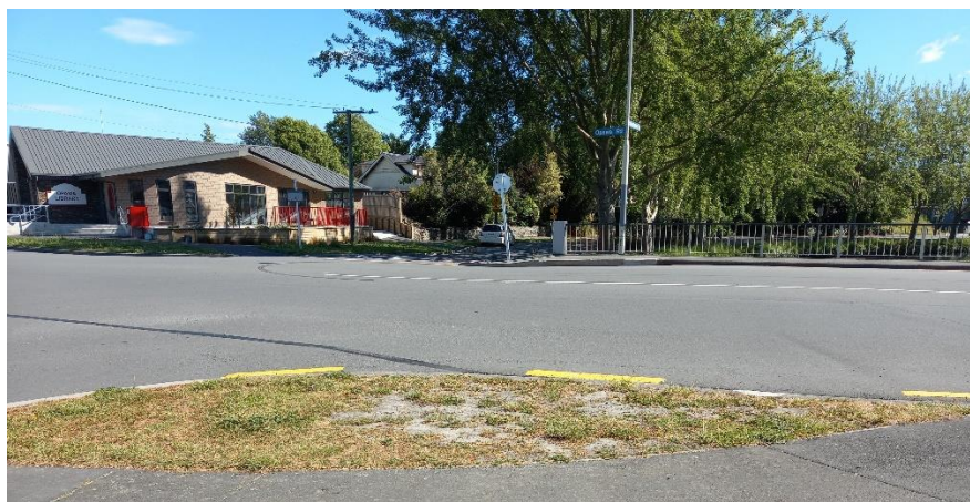
Figure 4: Crossing location of concern (west side of bridge)
