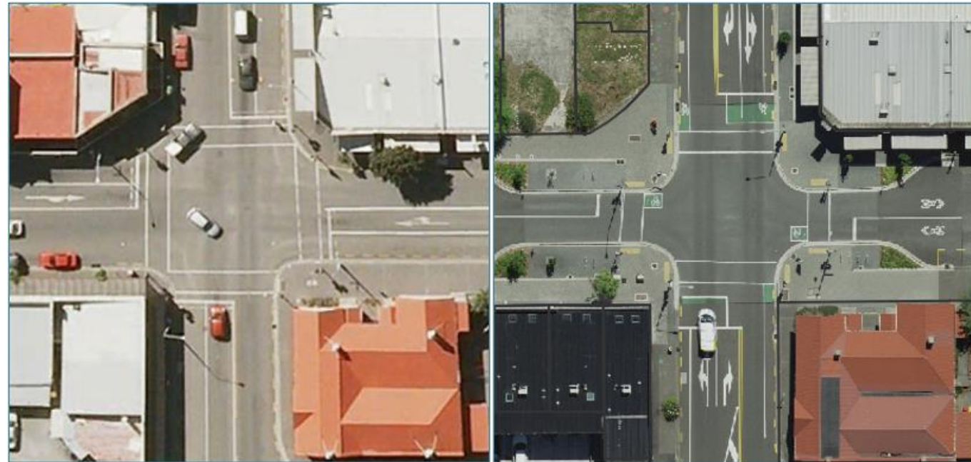
Worcester/Stanmore intersection, Christchurch
